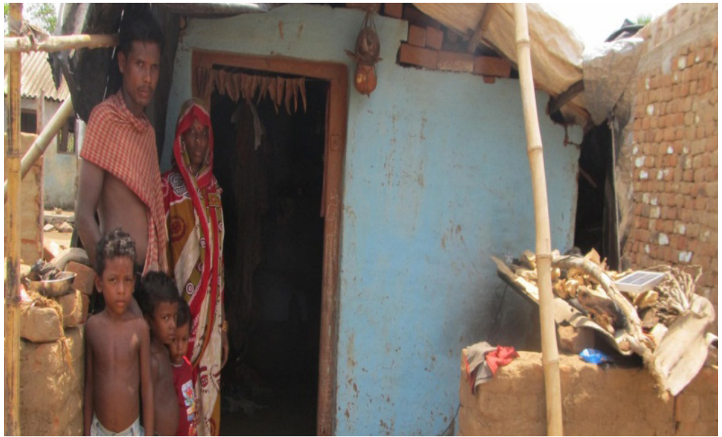
Janakin with her family at dilapidated house after cyclone
